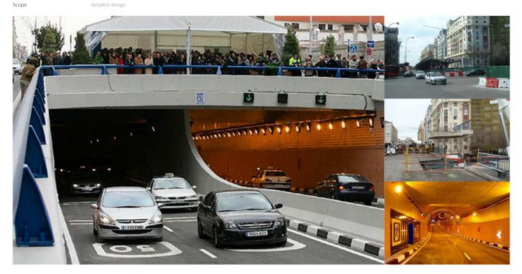
The subterranean roadway is composed of two independent twin tunnels which have two lanes in each direction, connected by emergency exits every 100m.
